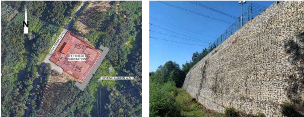
Figure 1 – Location of the existing gabion wall near the electrical substation.
